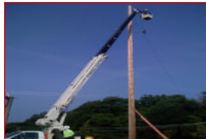
ISSUE #1 - Stansell Electric replaces the broken insulator.
